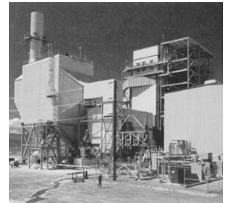
The Honey Lake Biomass & Geothermal Power Generation Plant.
